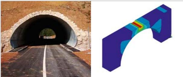
Fig. 2: Nonlinear stability analysis of a sheet metal tunnel construction
