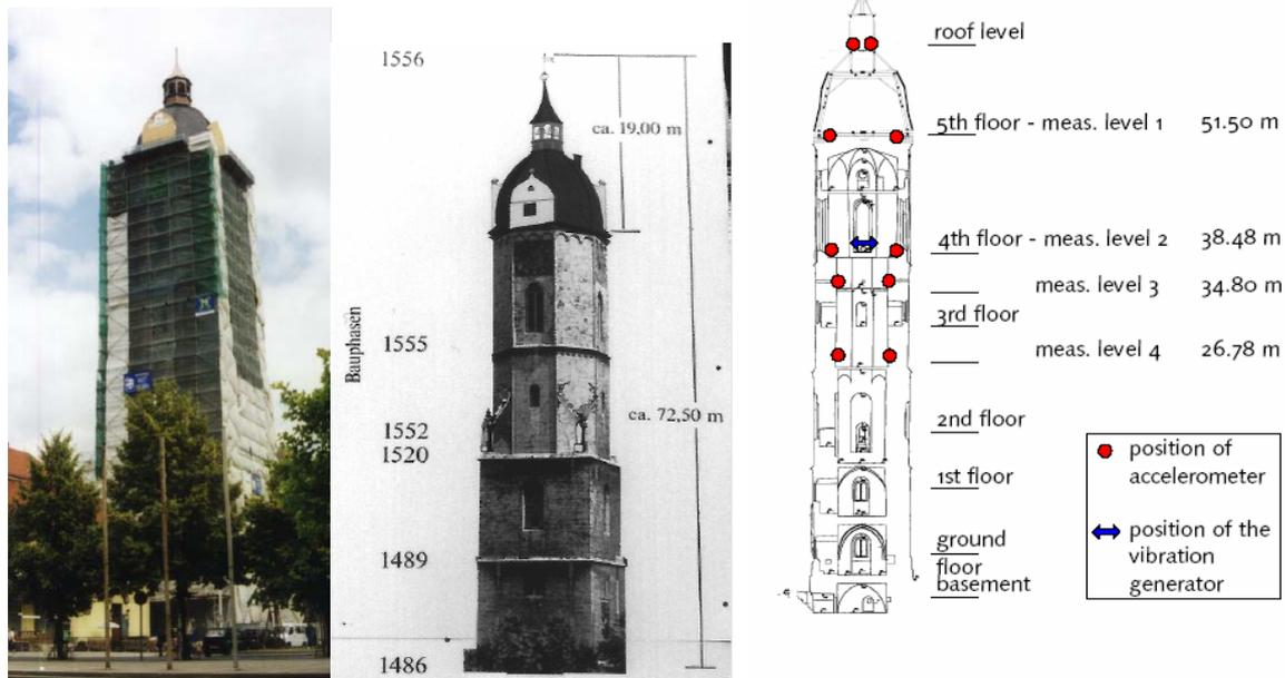
Fig. 2. Left – Bell tower during reconstruction, Middle – building history, Right – Positions of the vibration generator and the positions of the accelerometer.
